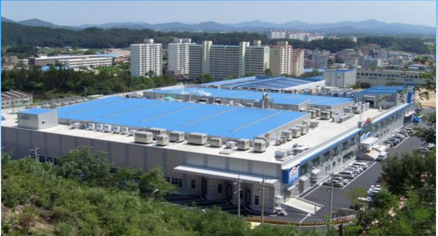
Electrical Work for Utility & Instant Rice Building in CJ Cheiljedang Food Production Station, Korea / Completion 2018
