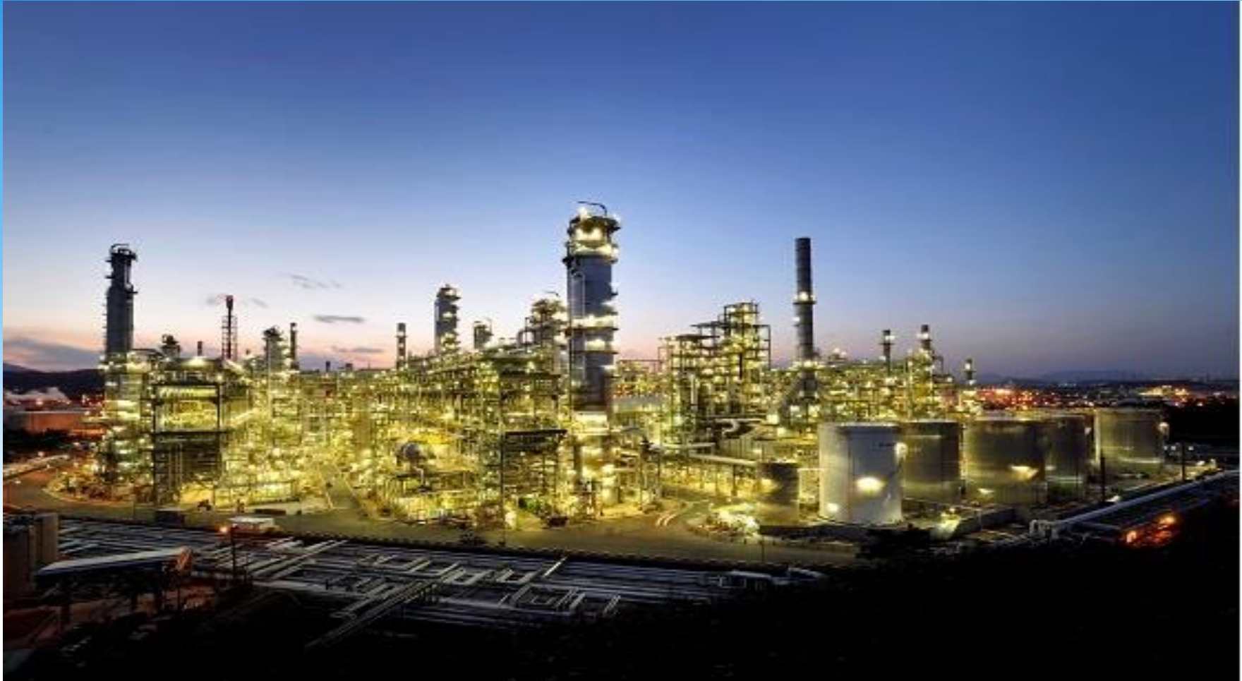
Electrical & Instrument Work for Low Pressure Steam Turbine Project in S-oil, Korea / Completion 2016
