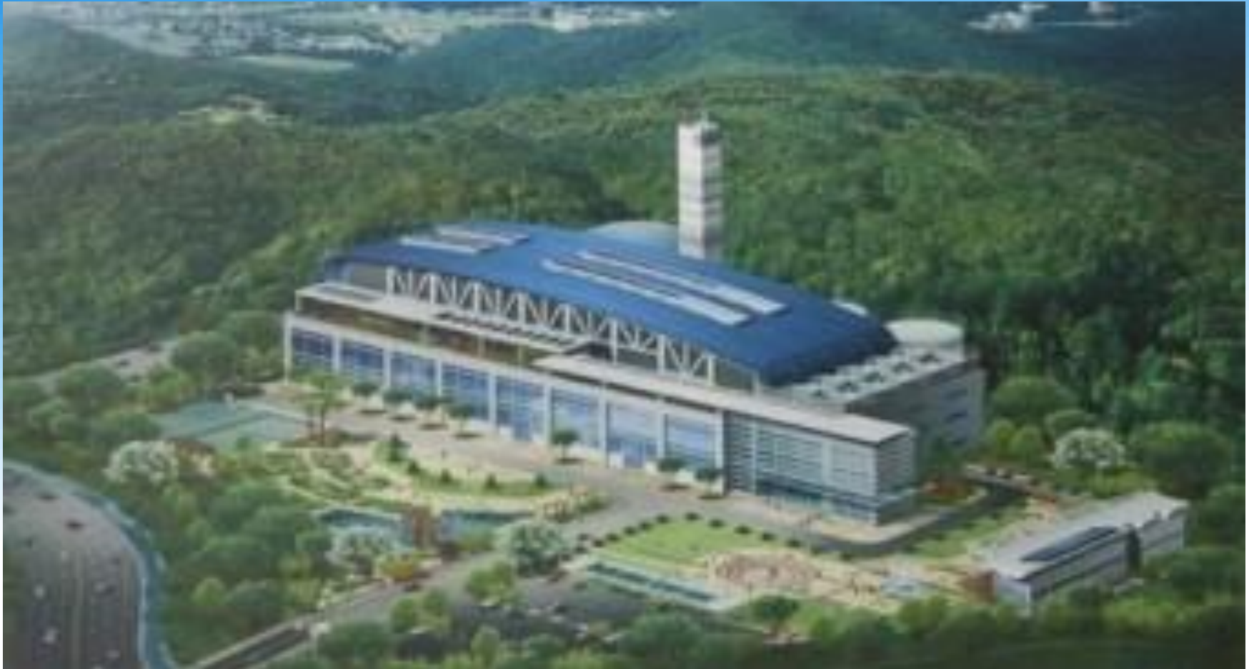
Instrumentation work construction of Yeosu natural Power Plant Korea / Completion 2023
