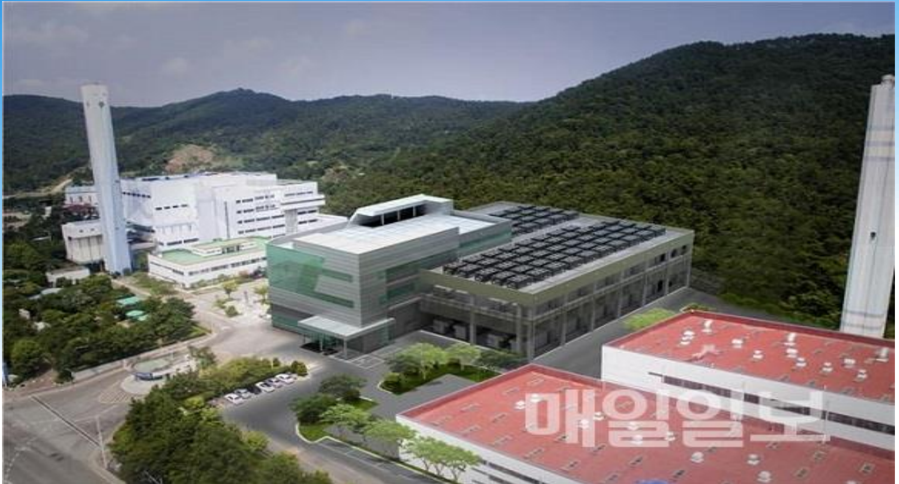
Electrical & Instrument Work for Buan Green Energy Electricity Generator Project, Korea / Completion 2017
