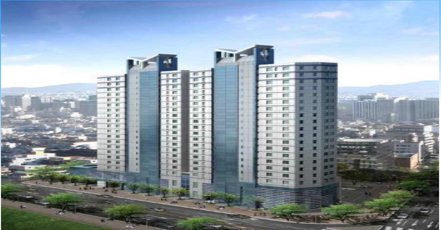
Electrical Work for SK Leaders View Office-tel in Yeoksam-dong Seoul, Korea / Completion 2014
