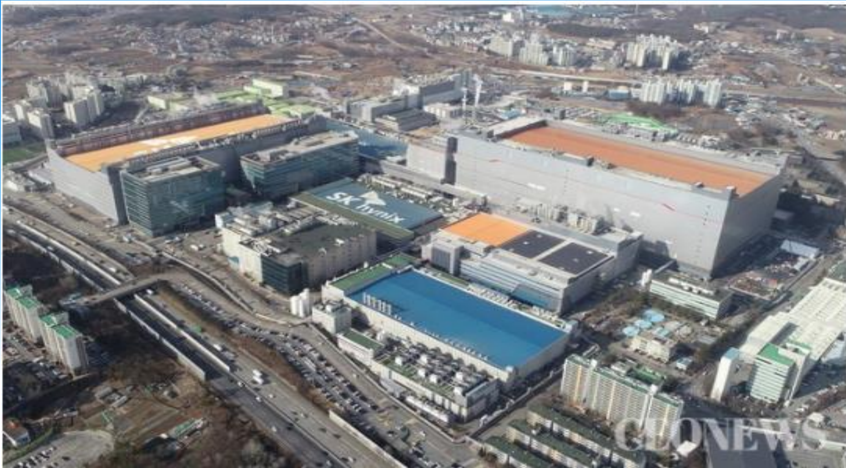
Electrical & Instrument Work for SK Hynix M16 Ph-1 Project Korea / Completion 2021
