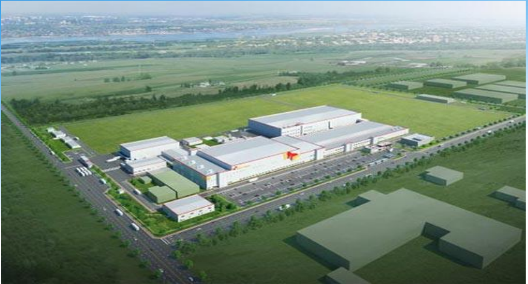
Electrical Work for Battery Cell Production Plant in SK Innovation Co., Korea / Completion 2017
