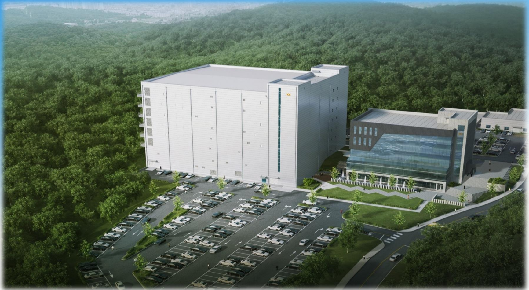
Telecommunication Work for #K8 Battery Building in SK Innovation Co., Korea / Completion 2018
