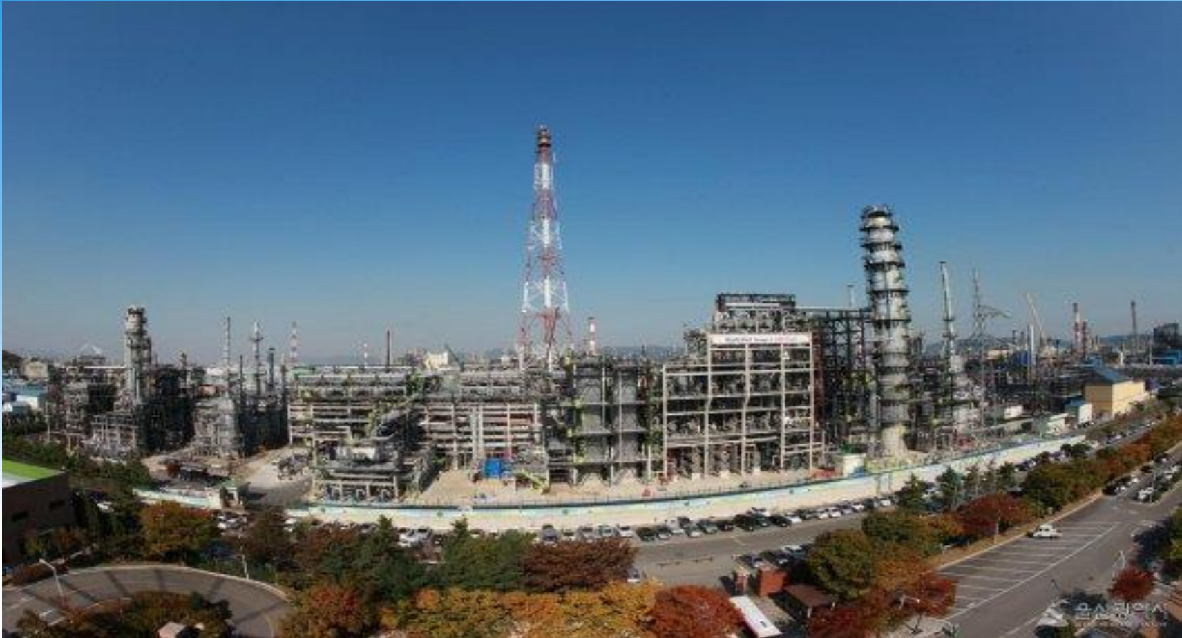
Electrical Work(B area) for S-Projct of SK Energy Co. Korea / Completion 2020
