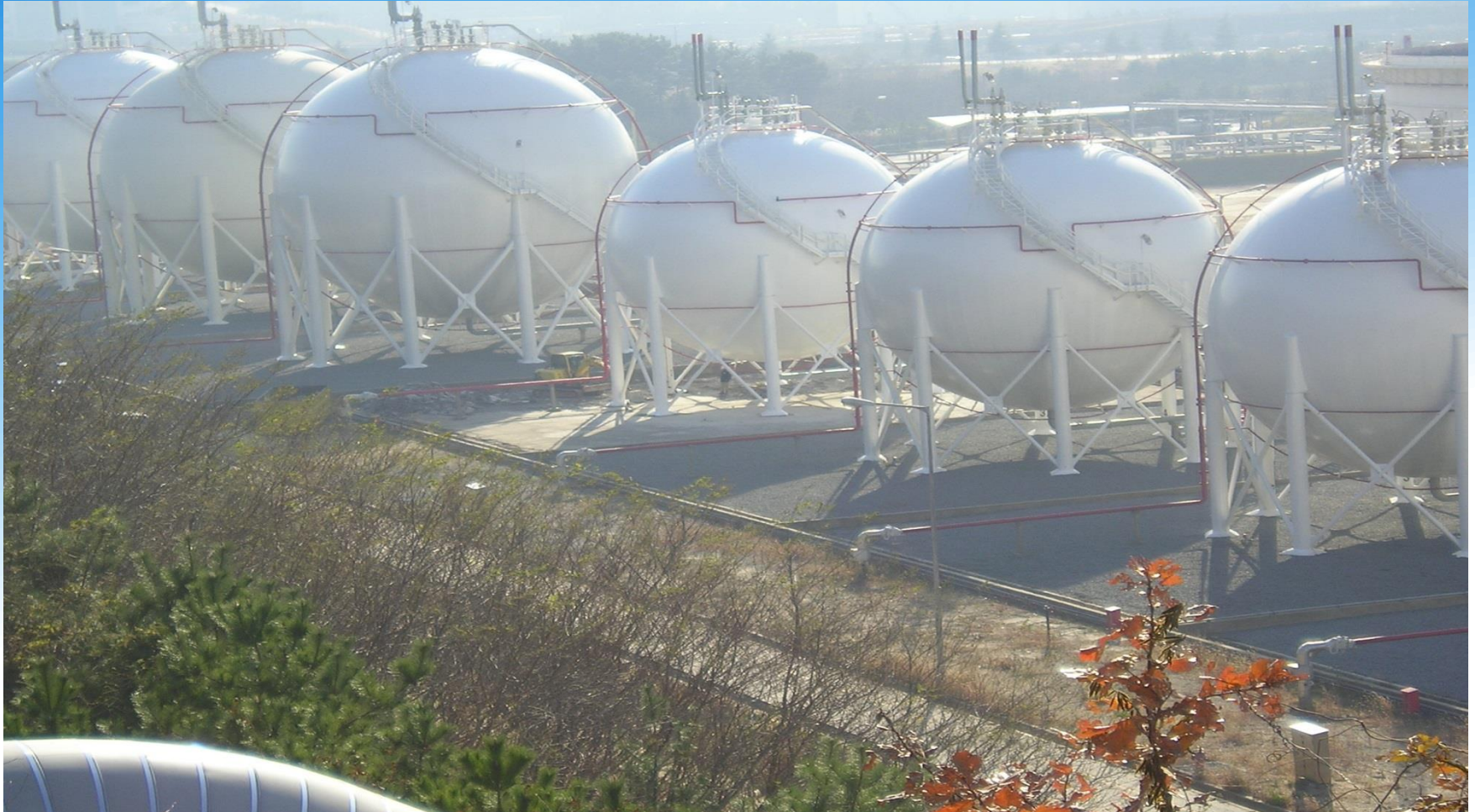
Electrical & Instrument Work for SK Gas Ulsan Ball Tank Station Korea / Completion 2018
