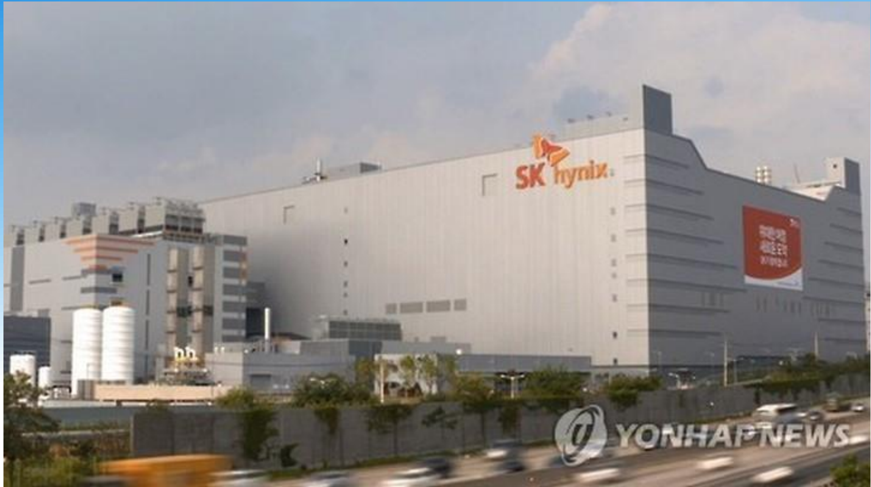
Electrical Work for SK Hynix M14 Ph-4 Project, Korea / Completion 2017
