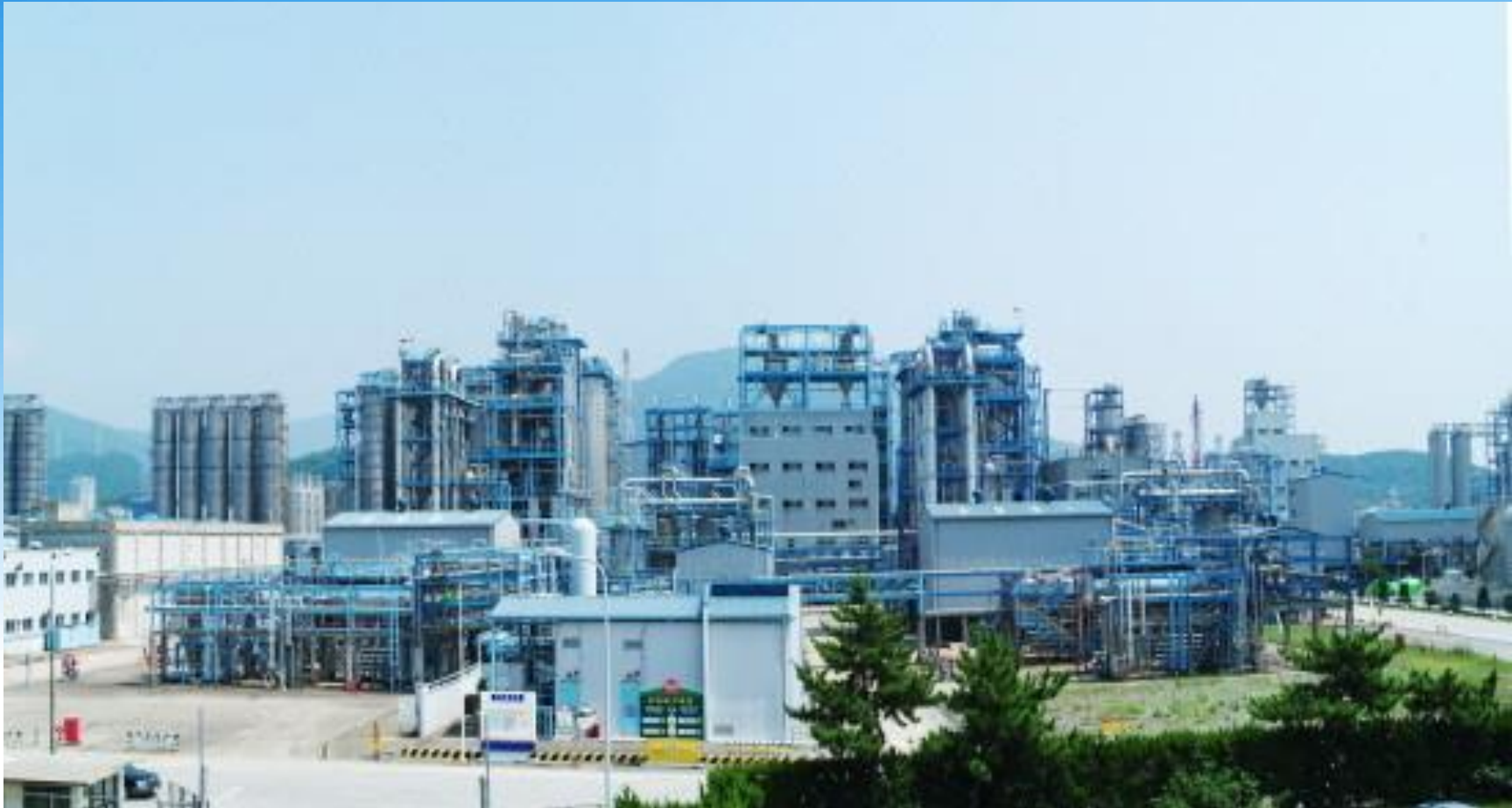
Electrical & Instrument Work for Ulsan PP Project Korea / Completion 2020
